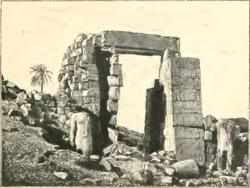
THE FIRST PYLON OF HARMHABÎ AT KARNAK. 1
